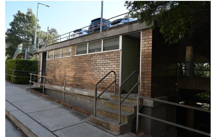
Wade Lane Gordon toilet block
